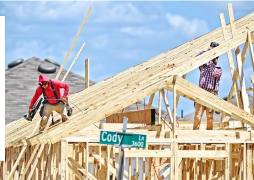
Construction workers frame a house Tuesday at the corner of Cody Lane and Doris Drive, in north Denton. A new state law limits what cities can do to regulate construction materials used by homebuilders.
