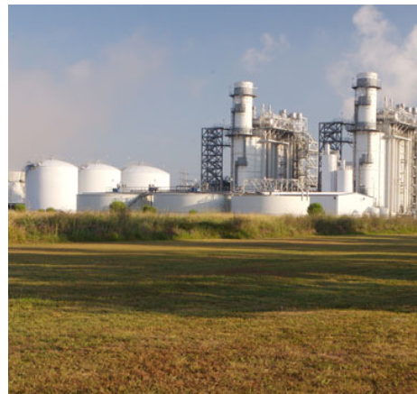
IMAGE: CALPINE'S JACK A. FUSCO ENERGY CENTER, © JIM OLIVE, 2008
